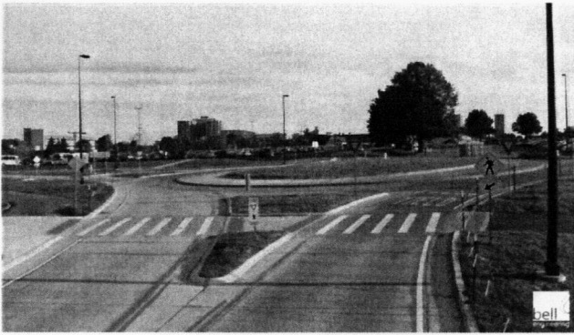
Alumni Drive Roadway Realignment
