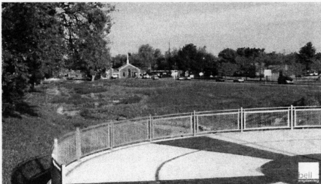
University of Kentucky FEMA Flood Mitigation Project
