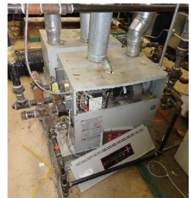
The existing boilers at Detention Center will be replaced with new boilers installed to maximize efficiency
