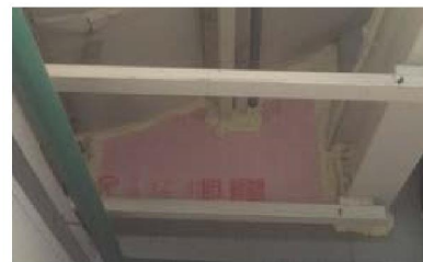
Example of the addition of insulated materials with foam sealant used to prevent uncontrolled air infiltration at KCTCS Owensboro.
