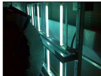
UV-C Light Installation at the Kentucky State Capitol Annex
