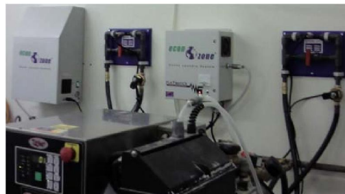
An ozone laundry system will be installed to reduce hot water requirements and protect linen life
