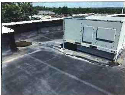
HVAC condensate drain needs to be extended. It is causing water ponding.
