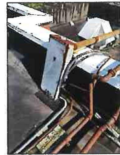
Panel sitting on ground with loose wires
