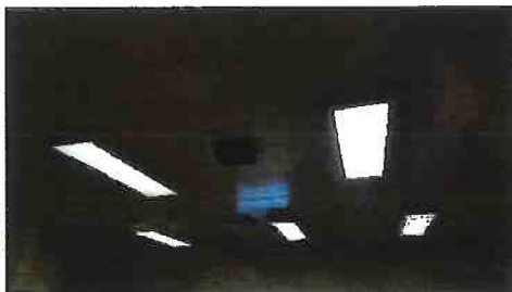
Cell secured T8 32 watt fixtures
