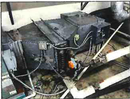
Aged Indoor Air Handler with poor wiring and duct runs
