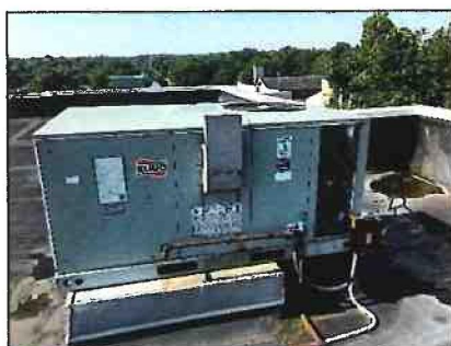
10 SEER RTU with R22 refrigerant
