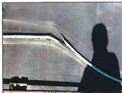
Electrical conduit splitting in multiple areas on the roof
