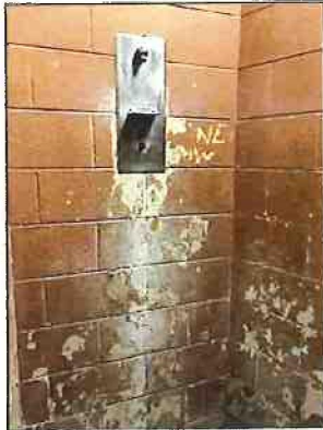
Shower head with Acorn Push Button timer
