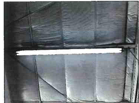
T-8 High Wattage Fluorescent Lighting in Truck Bay
