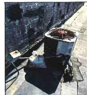
Aged Split System on the roof
