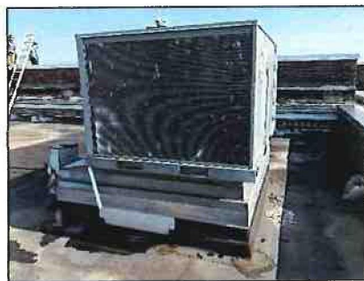
Unit with coil damage and poor drain
