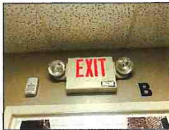
Some exits signs are LED and some are Incandescent
